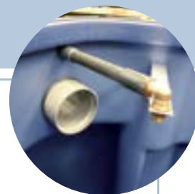
Detail of spray nozzle inside separator
