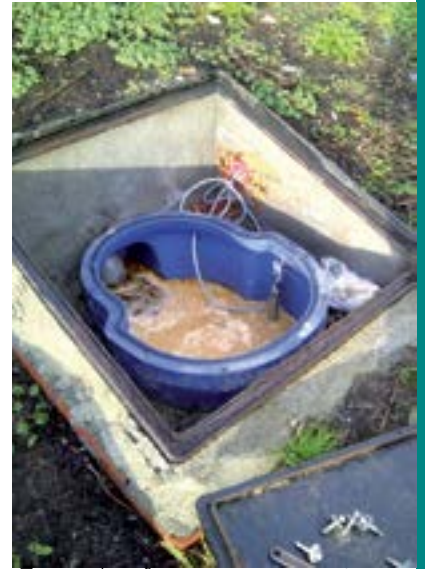
Example of a grease separator needing to be emptied
