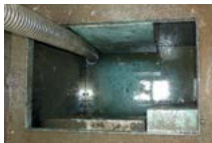
Draining the separator chamber
