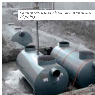
200 l/s steel oil separators near the Toulouse bypass (64)
