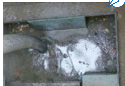
Resuspend settled sludge before pumping.
