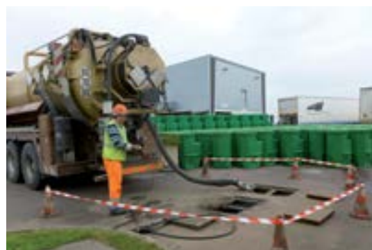
Resuspend settled sludge before pumping.
