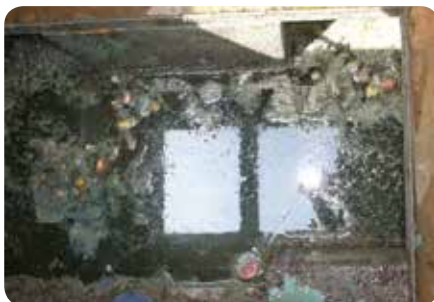
View of the sludge chamber
