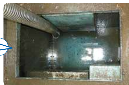
Emptying of the separator chamber
