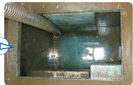
Emptying of the separator chamber
