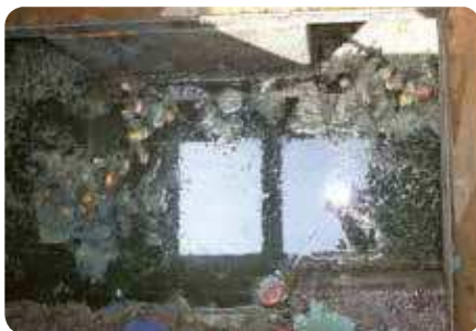
View of the sludge chamber
